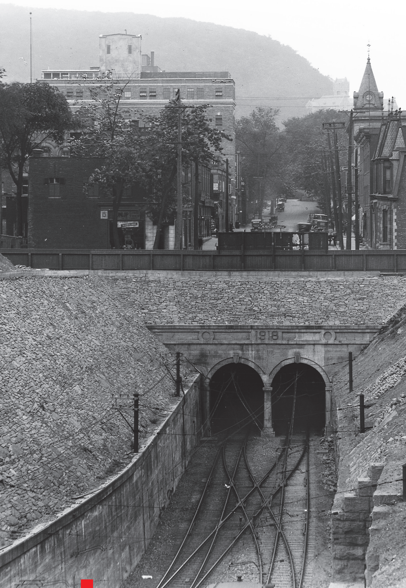
CNR tunnel under Mount Royal, Montréal, QC, 1918 (Ref 3).
